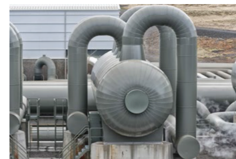
• the water supply pump station
